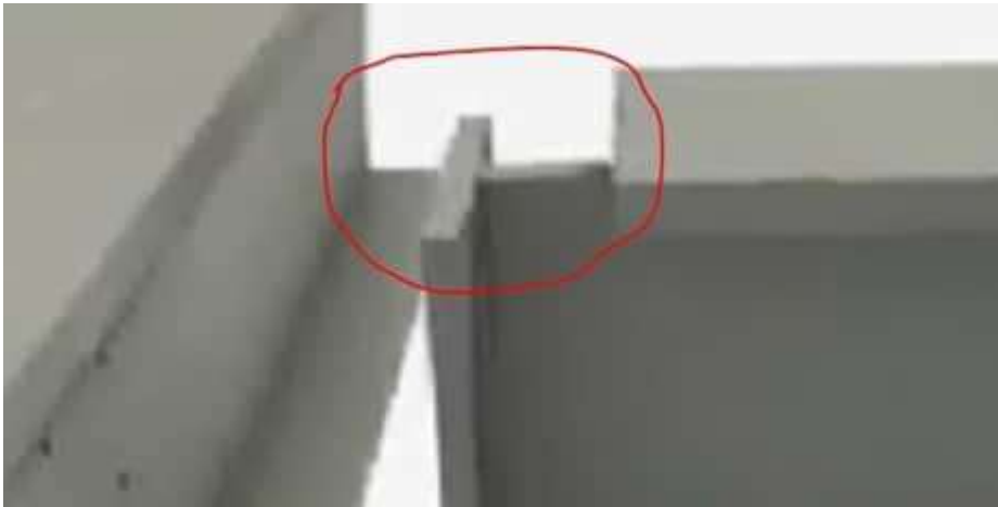
Notched Part of Secondary Beam
